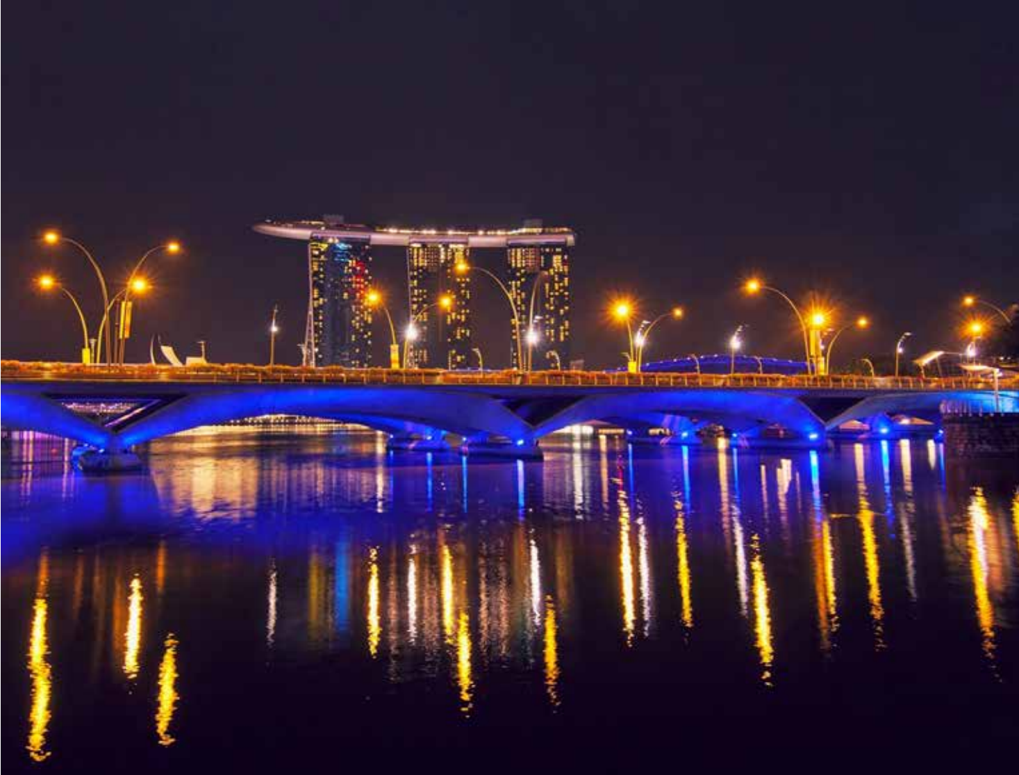
Bridge - Esplanade Bridge, Singapore
